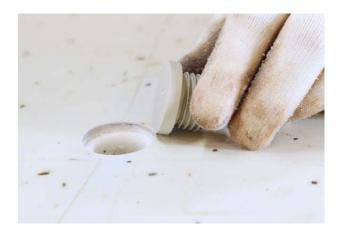
... drive it into the hole with a plastic hammer.
