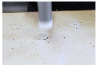
The remaining protrusion is removed easily with a paint remover and paint scraper. The plugs are made of polypropylene, just like the panel itself. Therefore future damage in the area of the plug can also be repaired easily using the extruder.
