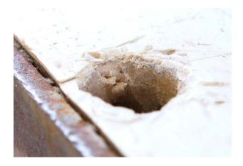
The aluminium repair cone is inserted into the tie hole as a shaper ...
