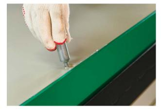
Once the panel has been aligned correctly, the rivet holes are drilled through the panel into the panel formwork. The panel is simultaneously countersunk using a  $120^{\circ}$  countersink (see page 9).
