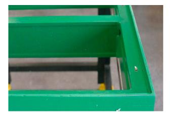
Although unnecessary for panel integrity, silicone may be gunned into the corner of the contact surface of the panel formwork to prevent concrete slurry entering the area between the formwork and the panel after installation.
