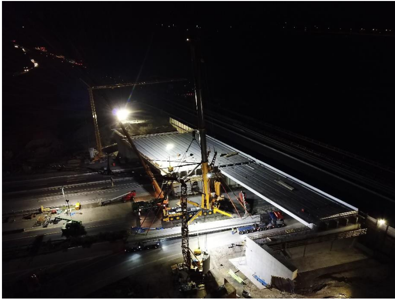
Construction of a temporary bridge at motorway junction Lotte/Osnabrück, © Rekers Betonwerk GmbH & Co. KG
