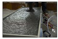
Casting with self-compacting concrete (SCC) – the system easily withstands the pressure acting on the formwork.
