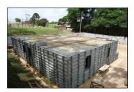
The procedure is always the same: initial assembly of the internal wall formwork, installation of blockouts, placement of concrete reinforcement and integration of electrical and water ducting.
