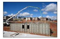
The slab formwork is installed and cast after assembly of the outer wall formwork. The wall and ceiling thicknesses vary between 10 and 20 cm and 8 and 15 cm respectively.
