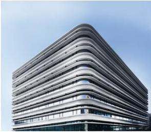
In total, 1,150 finished parts were made with 13 formwork panels. This is the theoretical equivalent of 88 finished parts for each formwork panel. And that with consistently good finishes from the first to last piece.
