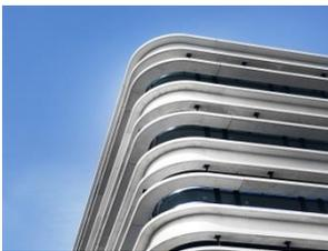
The façade is made up of the thermal shell and curtain-type concrete sections. The benefit: the sections also create their own high levels of shade so there was no need to install additional sun shading.
