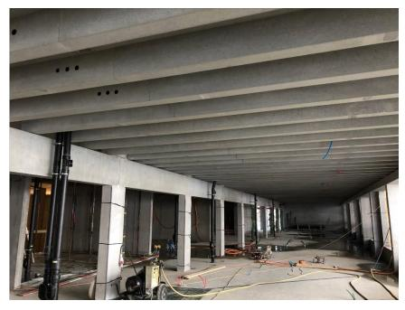
The T-beam ceiling panels in the new "M" ward block of the Chur cantonal hospital.  $\ensuremath{\mathbb{C}}$  alkus AG
