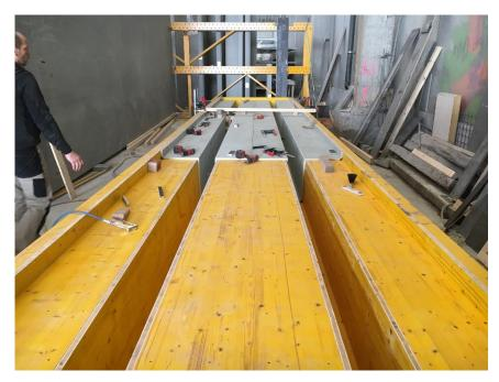
The wooden construction for the12 metre-long T-beam ceiling panels is covered with alkus® solid plastic panels. © alkus AG
