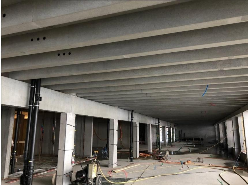
The T-beam ceiling panels in the new “M” ward block of the Chur cantonal hospital. © alkus AG
