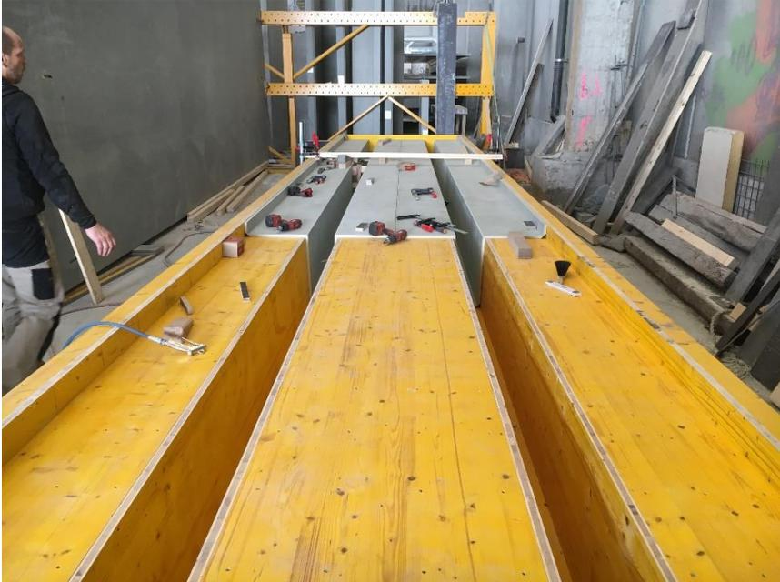
The wooden construction for the 12 metre-long T-beam ceiling panels is covered with alkus<sup>®</sup> solid plastic panels. © alkus AG
