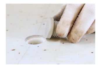
... drive it into the hole with a plastic hammer.
