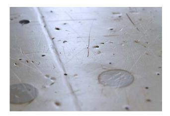
Protrusions of nail holes and minor soilings can also be removed quickly and easily with the paint scraper.
