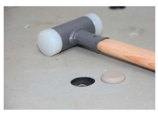
Insert repair patch (see page 9) and drive it into the hole with a plastic hammer.
