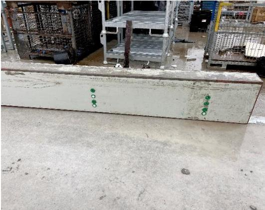
After 10 uses: The alkus<sup>®</sup> formwork panel with the alkus<sup>®</sup> sealing cones in the Peri formwork system. | © Bold GmbH & Co KG
