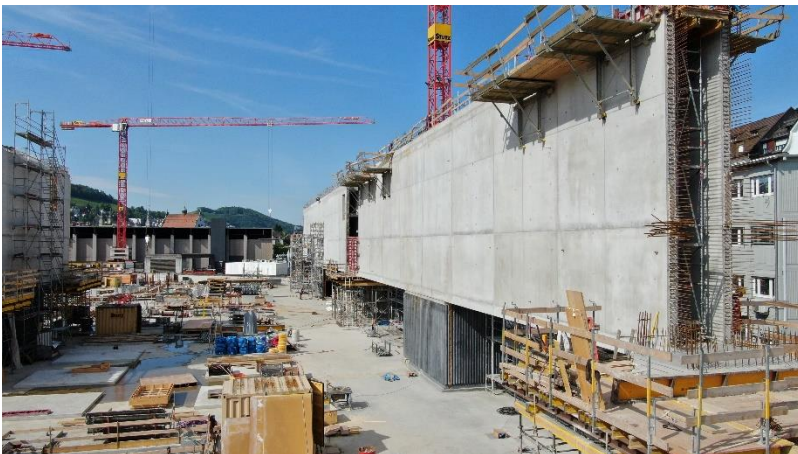
Core structure of the new Olma hall 1. | © alkus AG
