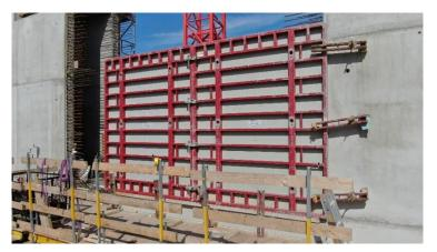
Use on site: The alkus $^{\ensuremath{\mathbb{S}}}$  solid plastic panel in a PERI formwork system. |  $\ensuremath{\mathbb{C}}$  alkus AG
