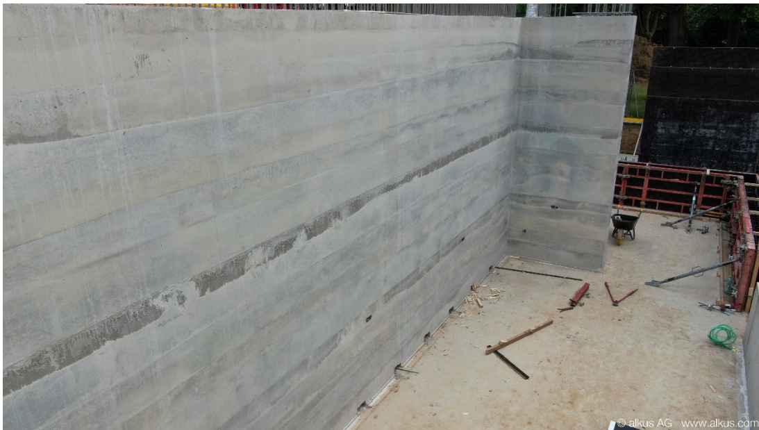
Figure 1: Spectacular wall without gaps and anchor tie holes.
