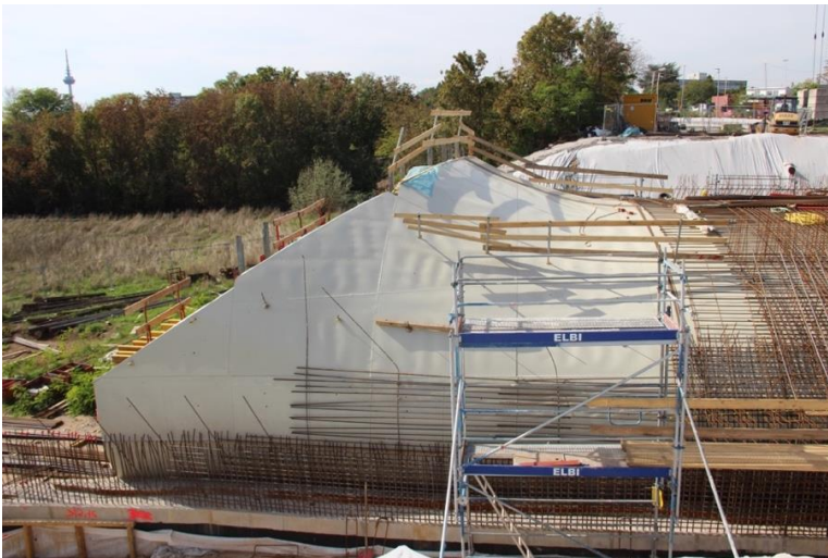
The alkus ® SF Flex - suitable for particularly demanding projects in special formwork construction and is available in 3, 4 and 5 millimeter thicknesses. | © Kiefer Schalungsbau GmbH
