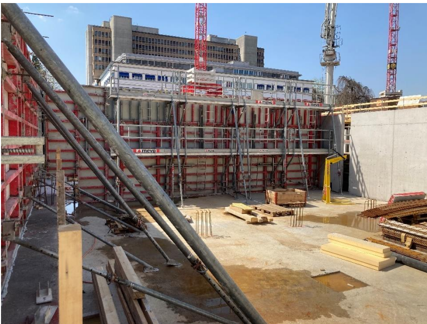
MEVA Mammut 350 wall formwork covered with the alkus ® solid plastic panel. | © MEVA
